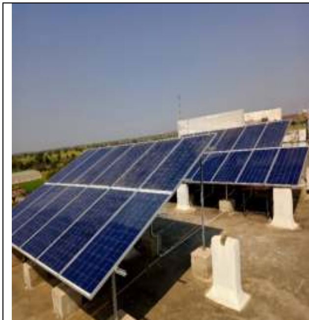
Fig5: Solar PV Plant of 8 kw installed in the roof of building
